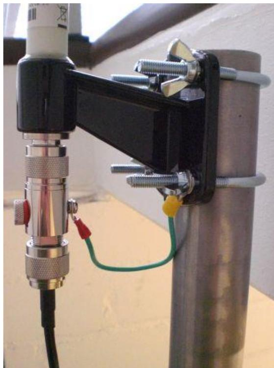
Figure 9: Assembling the antenna with the lightning protection system
